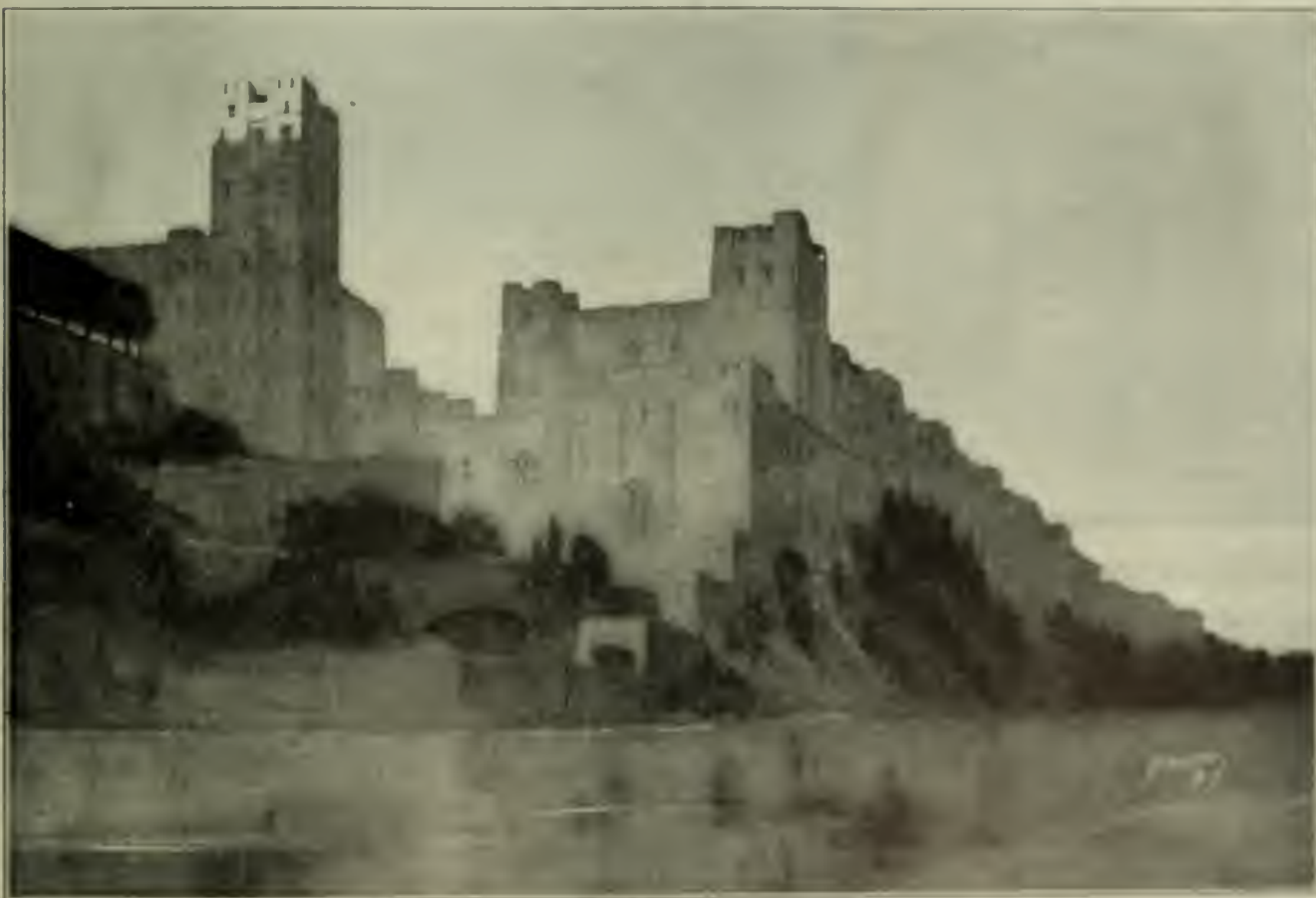
FIG. 1. THE WEST POINT POWER HOUSE, BUILT BY THE BUREAU OF REVENUE IN 1887
